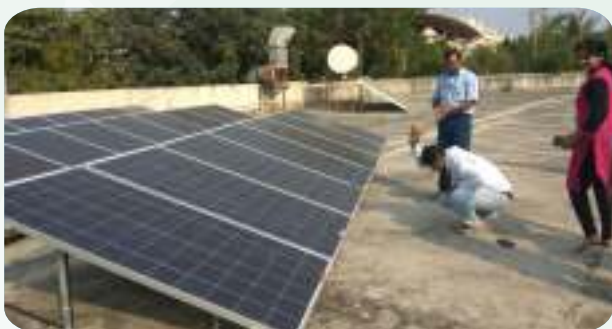
Installation of 8KW Grid Tied Solar Power Plant
