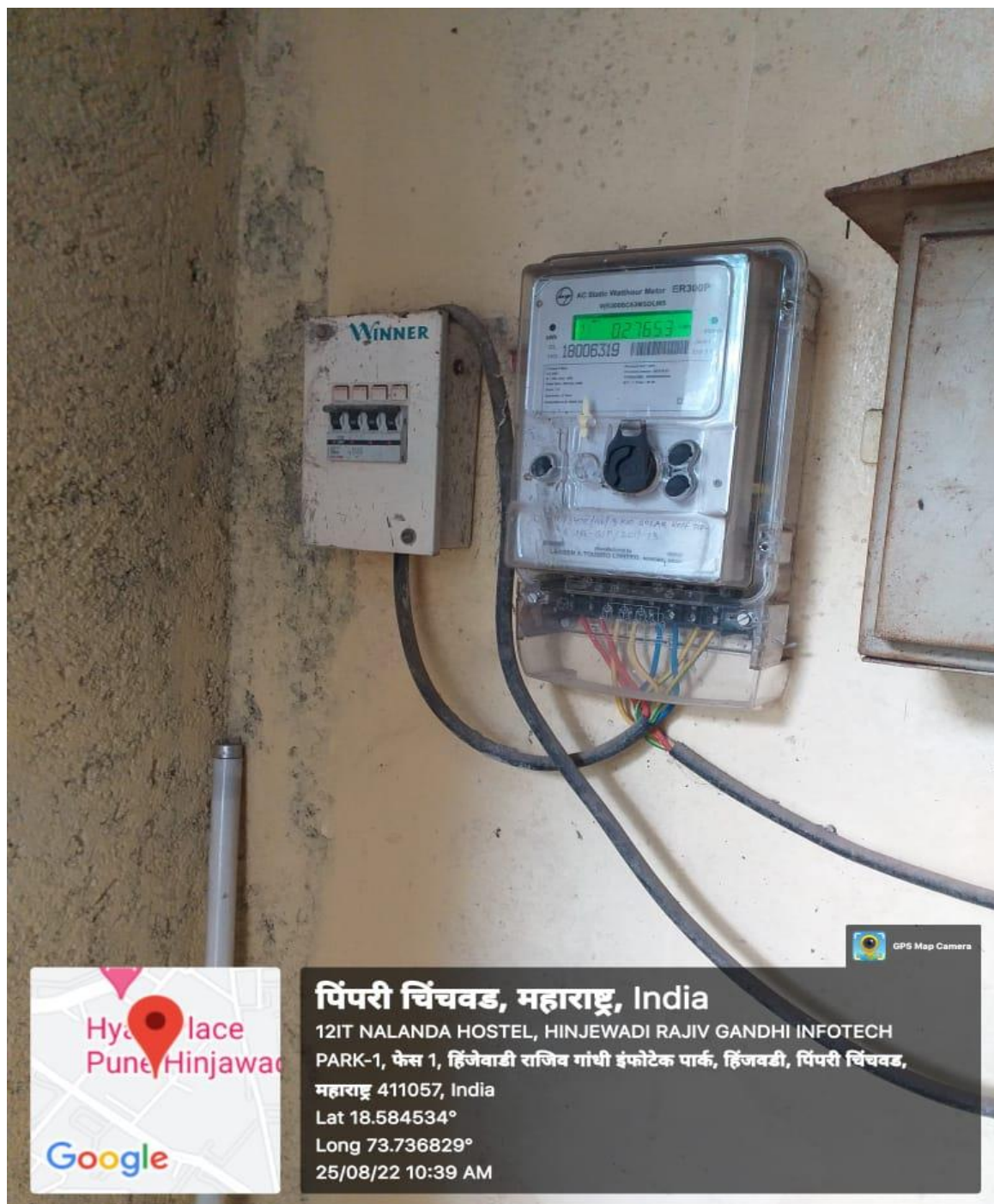
Grid connection of solar panel installation (Net metering)
