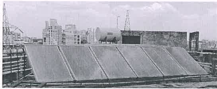
Figure 5.2 : Photograph of solar thermal hot water system
