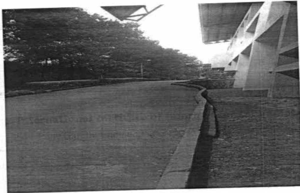
Approach road towards Ramp-2 and view of college building
