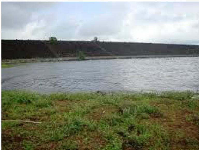
The team visited the dam on 3<sup>rd</sup> January in the evening at 4:30 pm. This dam is an earthen dam. It's total length is 1215 meter, and it's foundation height is 36 meters. The purpose of building this dam was to bring the surrounding land under water and irrigation. We enjoyed the sunset at the dam.
