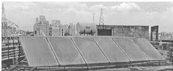
Figure 5.2 : Photograph of solar thermal hot water system
