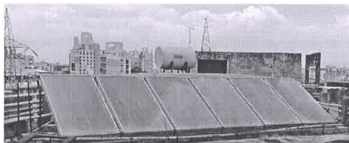
Figure 6.2 : Photograph of solar thermal hot water system
