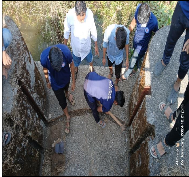
Photo 2: Cleaning of KT Weirs Slots
